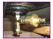
The water exit hole on the side of the auto drain valve is aimed straight down, so you can't see it very well. If you look carefully at the <u>enlarged image</u>, you can just make out the edge of it on the bottom of the valve.
